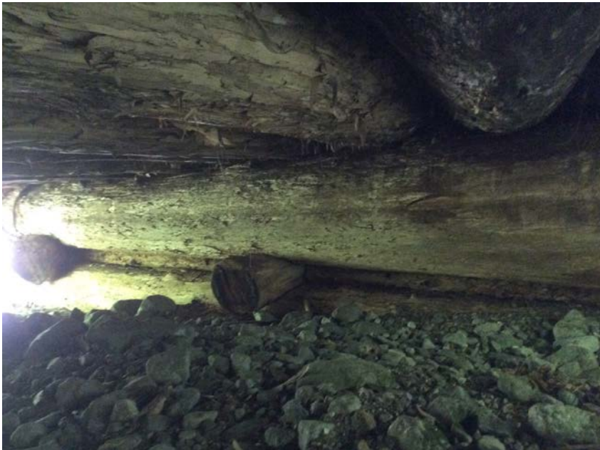
Right Bank Abutment when facing downstream
