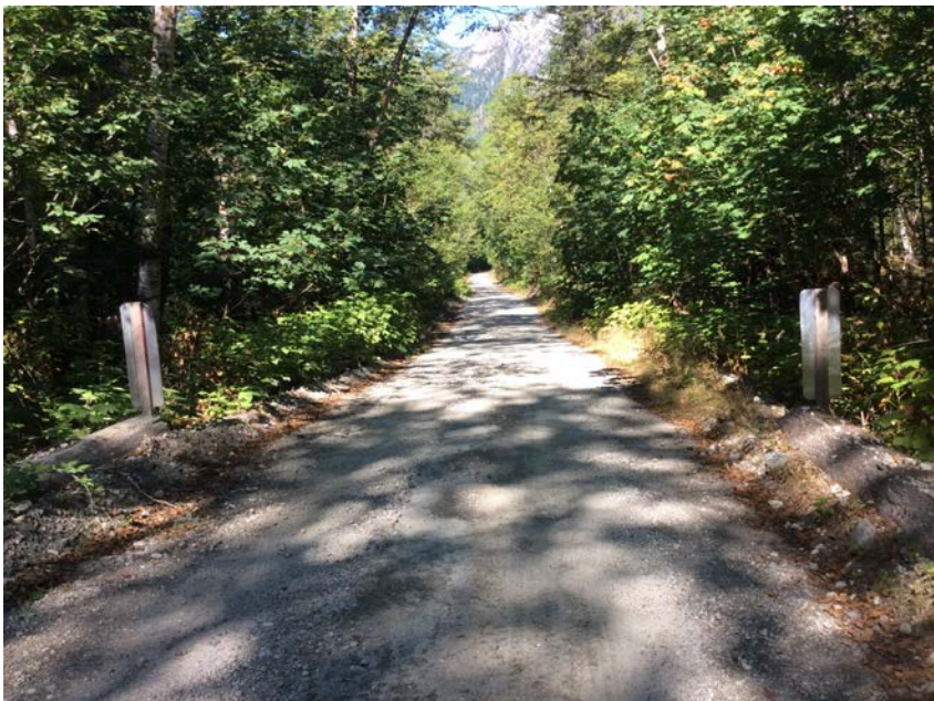
Right approach viewed from bridge
